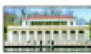
Project Park Alliance is planning an urban restoration of the Audubon Center on weekends so it can use the historic building as a park on the weekends.
